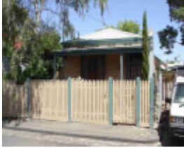
richmond tyson street richmond tyson street 10
