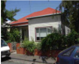
richmond tyson street richmond tyson street 12
