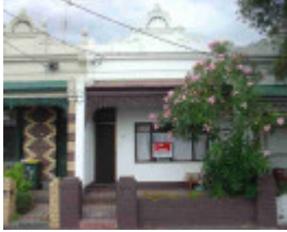
carlton north station street carlton north station street 616
