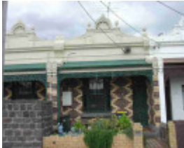
carlton north station street carlton north station street 618
