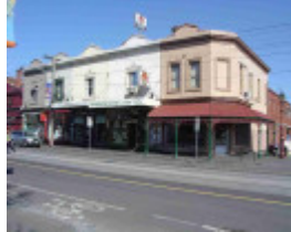
Fitzroy Brunswick Street 403- 411.JPG
