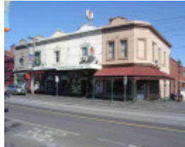
Fitzroy Brunswick Street 403- 411.JPG
