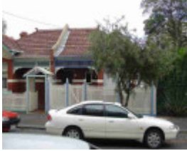
richmond sherwood street richmond sherwood street 24
