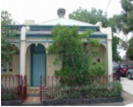
carlton north station street carlton north station street 210
