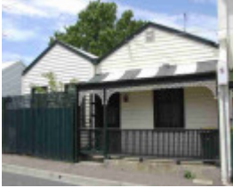
richmond tyson street richmond tyson street 5-3
