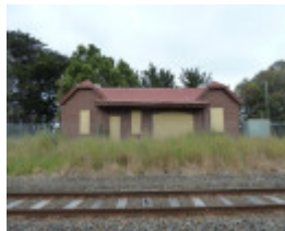
H1584 PIRRON YALLOCK RAILWAY STATION COMPLEX LHA 2015 1.JPG
