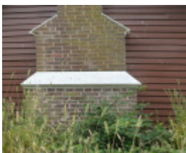
H1584 PIRRON YALLOCK RAILWAY STATION COMPLEX LHA 2015 3.JPG
