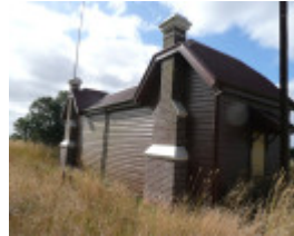
PIRRON YALLOCK RAILWAY STATION COMPLEX SOHE 2008
