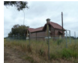
H1584 PIRRON YALLOCK RAILWAY STATION COMPLEX LHA 2015 2.JPG
