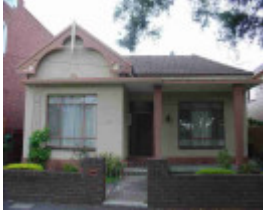
clifton hill heidelberg road clifton hill heidelberg road 35
