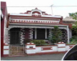
abbotsford trenerry crescent abbotsford trenerry crescent 3
