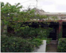
abbotsford trenerry crescent abbotsford trenerry crescent 5
