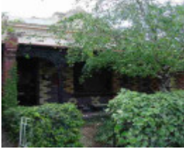
abbotsford trenerry crescent abbotsford trenerry crescent 7
