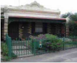
abbotsford trenerry crescent abbotsford trenerry crescent 11
