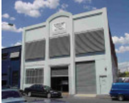
richmond wangaratta street richmond wangaratta street 51
