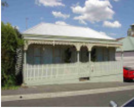
richmond waverley street richmond waverley street 3
