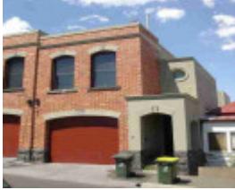
richmond waverley street richmond waverley street 9a
