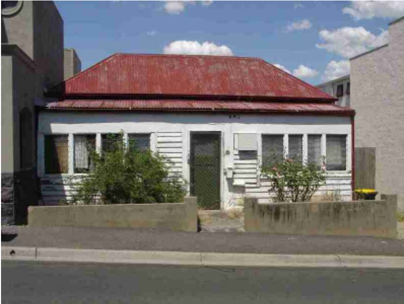
richmond waverley street richmond waverley street 11
