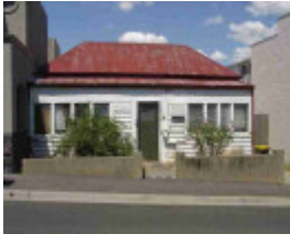
richmond waverley street richmond waverley street 11
