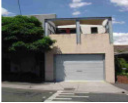
richmond waverley street richmond waverley street 13a
