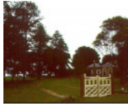
Point Cook Homestead Gates Side Facade July 01
