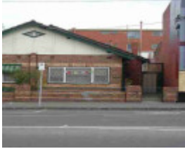
collingwood wellington street collingwood wellington street 347a
