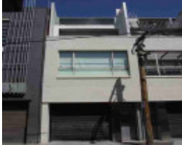
richmond wangaratta street richmond wangaratta street 28
