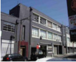
richmond wangaratta street richmond wangaratta street 30
