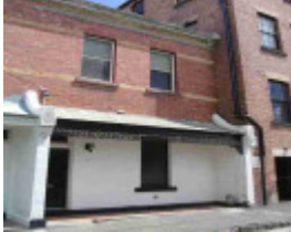
richmond waltham place richmond waltham place 12
