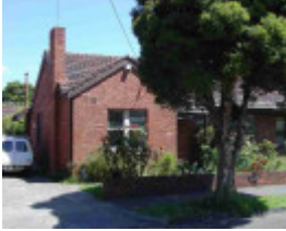
burnley westbank terrace burnley westbank terrace 24
