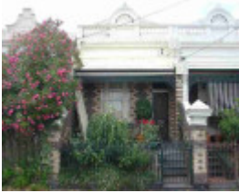
carlton north station street carlton north station street 560
