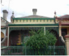
carlton north station street carlton north station street 569
