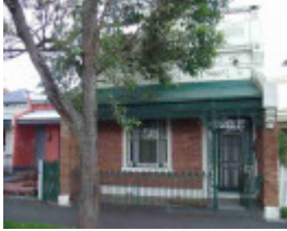
clifton hill heidelberg road clifton hill heidelberg road 61
