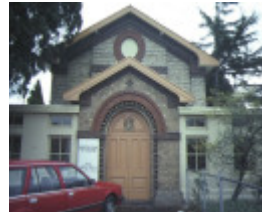
1 port melbourne courthouse policew station & lock up bay street port melbourne front view courthouse
