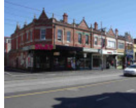
Fitzroy Brunswick Street 377- 387.JPG
