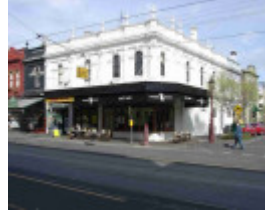
Fitzroy Brunswick Street 227- 233.JPG
