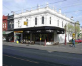
Fitzroy Brunswick Street 227- 233.JPG
