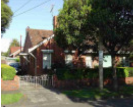
burnley tudor street burnley tudor street 13
