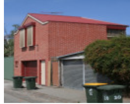
Rear of 16 Grant Street
