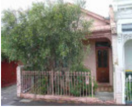
carlton north station street carlton north station street 282
