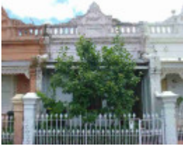
carlton north station street carlton north station street 387
