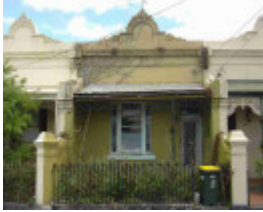
carlton north station street carlton north station street 393
