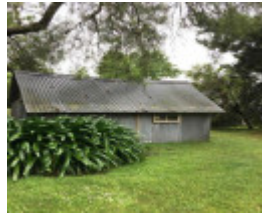
Outdoor toilet (2017).jpg
