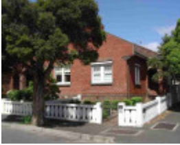
richmond waltham street richmond waltham street 20
