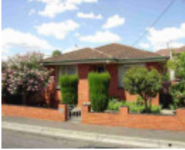
richmond wangaratta street richmond wangaratta street 9
