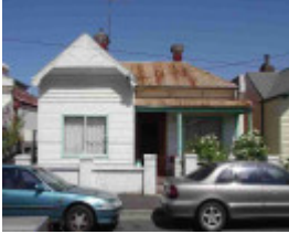
richmond wangaratta street richmond wangaratta street 10
