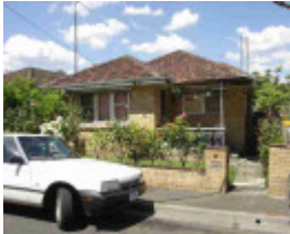
richmond wangaratta street richmond wangaratta street 11
