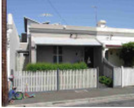
richmond wangaratta street richmond wangaratta street 14
