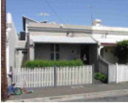
richmond wangaratta street richmond wangaratta street 14
