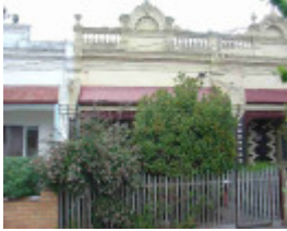
Carlton North Station Street 402.JPG
