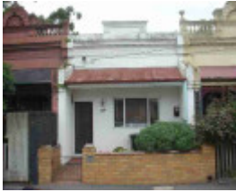
carlton north station street carlton north station street 404
