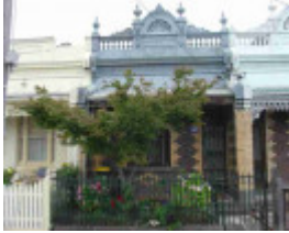
carlton north station street carlton north station street 416
