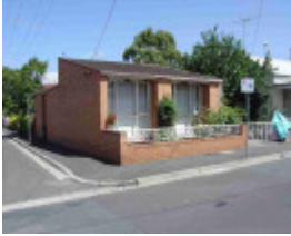
richmond woodlawn street richmond woodlawn street 10
