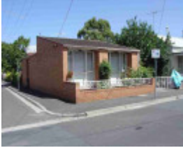
richmond woodlawn street richmond woodlawn street 10
