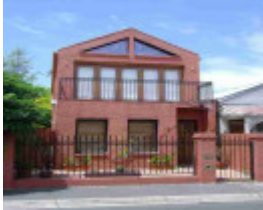
richmond woodlawn street richmond woodlawn street 15
