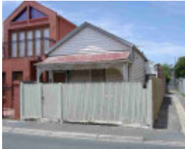
richmond woodlawn street richmond woodlawn street 17
