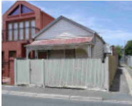
richmond woodlawn street richmond woodlawn street 17
