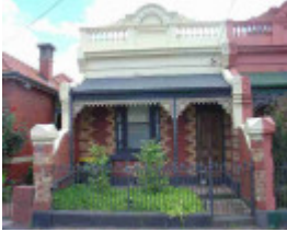
carlton north station street carlton north station street 451
