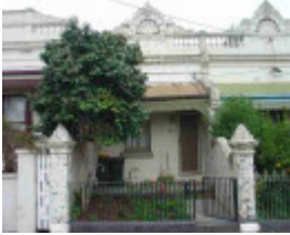
carlton north station street carlton north station street 464
